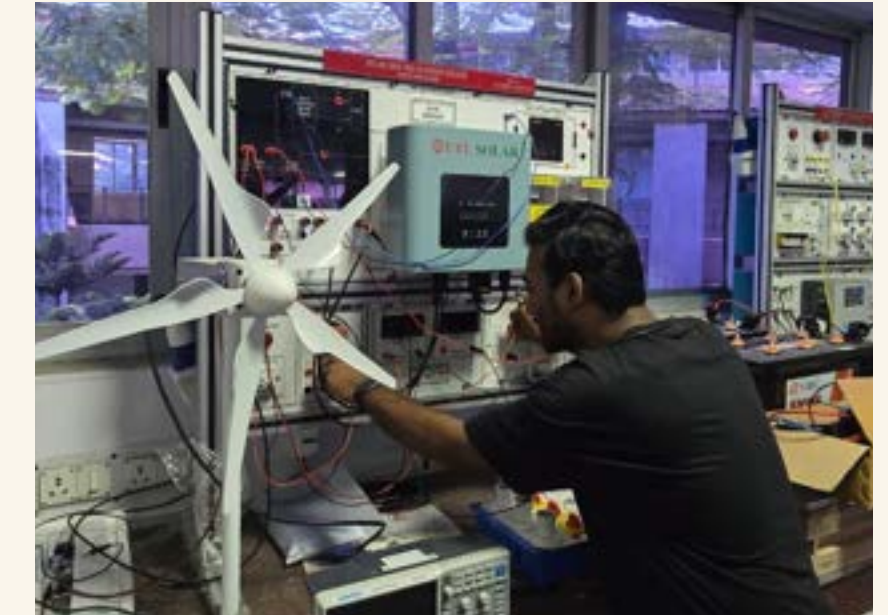
Smart Microgrid Laboratory
